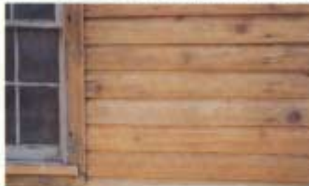
Up close: clean wood on the shed's siding (left) contrasts with peeling paint on the window frame (covered during removal). Steel water tank after partial cleaning—gray area shows no residual paint (below).
